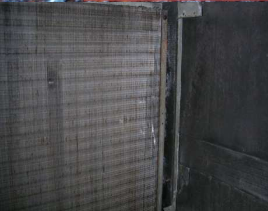
Various Infected Coils & Drain Pans
